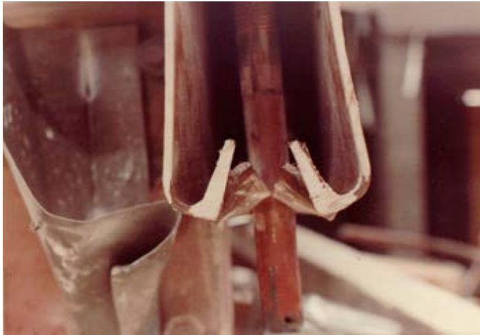
Close-up of one of the fourth floor beams.
