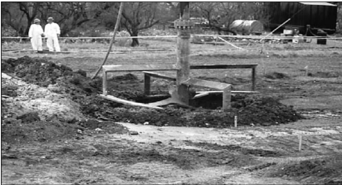
In situ mixing process with modified augers 1
