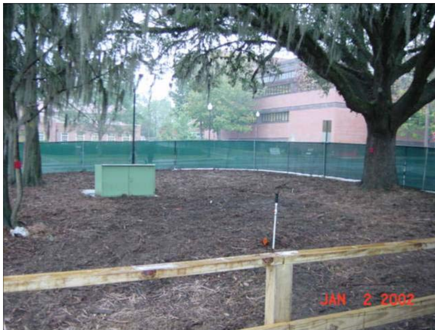
Constructed Fence for tree protection
