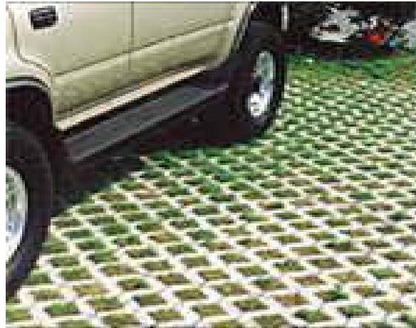
Turfblock parking lot
