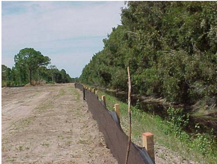
Installed – and not damaged – silt fence
