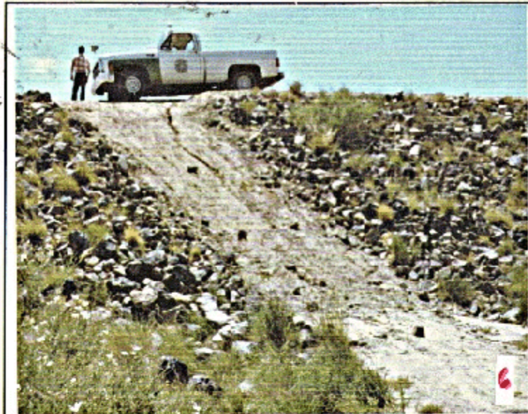
Photo 20. Everyone gets in. Riprap removed.
