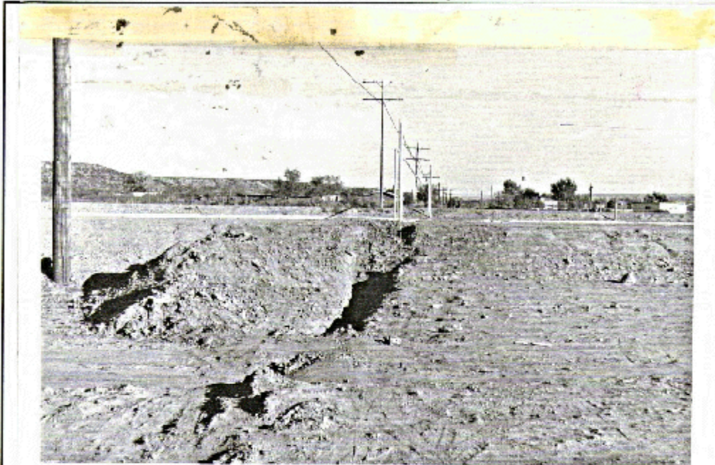
Photo 12. Unauthorized utility crossing
