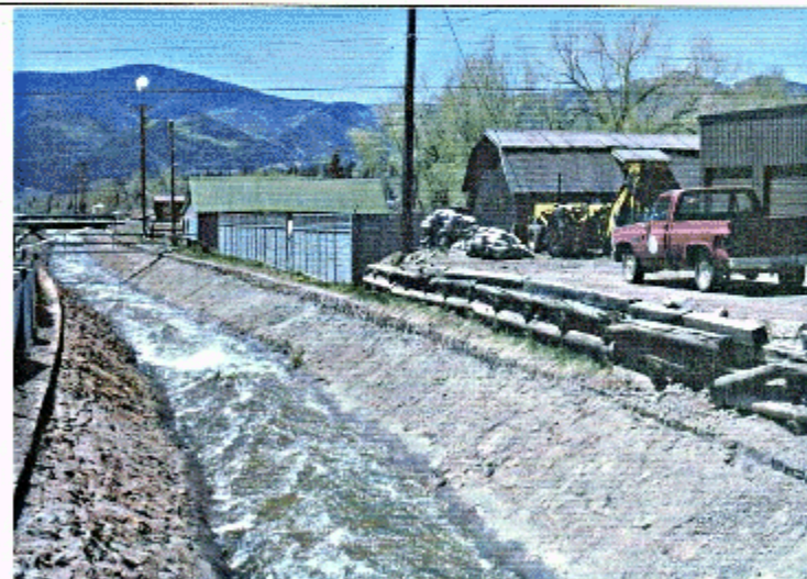
Photo C-18. Ready for Sandbagging, 1998
