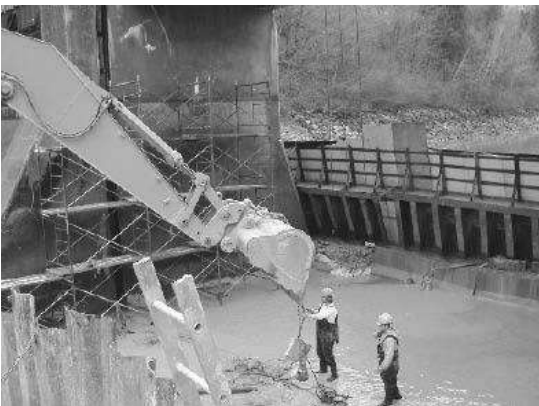
Figure 1.2. Bad weather slows dam construction.
