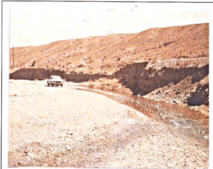
Photo 2.2. Levee erosion
