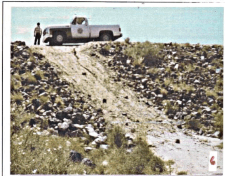
Photo 9.4. Riprap removed
